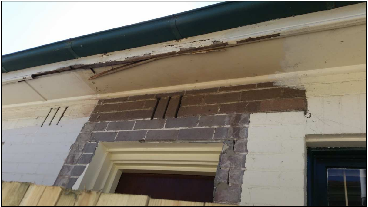
Photograph 3. 5 Station St, presumed asbestos eaves and paint in poor condition.
